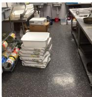
The new pizzeria's 1900 square floor of new concrete was swept scrupulously clean and dried prior to the applications of a 30 mils depth of product. Ecodur has almost double the adhesion of conventional epoxy coatings and readily permanently infills cracks and crevices. Uniquely, this plasticized gypsum can re-bond to itself if touch ups are required at any time during the lifetime of the coating can, in ideal conditions, be an almost indefinite period as the product does not shrink or crack.
