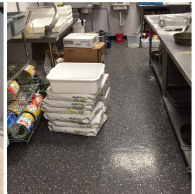
The new pizzeria's 1900 square floor of new concrete was swept scrupulously clean and dried prior to the applications of a 30 mils depth of product. Ecodur has almost double the adhesion of conventional epoxy coatings and readily permanently infills cracks and crevices. Uniquely, this plasticized gypsum can re-bond to itself if touch ups are required at any time during the lifetime of the coating can, in ideal conditions, be an almost indefinite period as the product does not shrink or crack.
