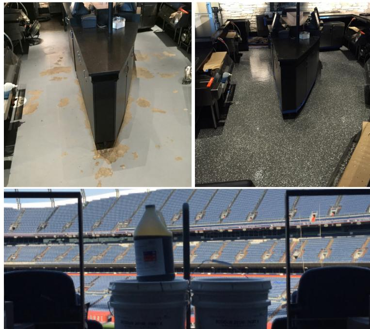
A major surface preparation had to be done prior to coating which included degreasing of food and beverage waste. The old, failing coating had to be completely removed and the surfaces left dry and absolutely clean. The restricted window for completion required fine planning and execution. The stadium has events all the time. Not completing the job on time was not an option as the VIP Club level brings in \$100,000s per day in sales.
